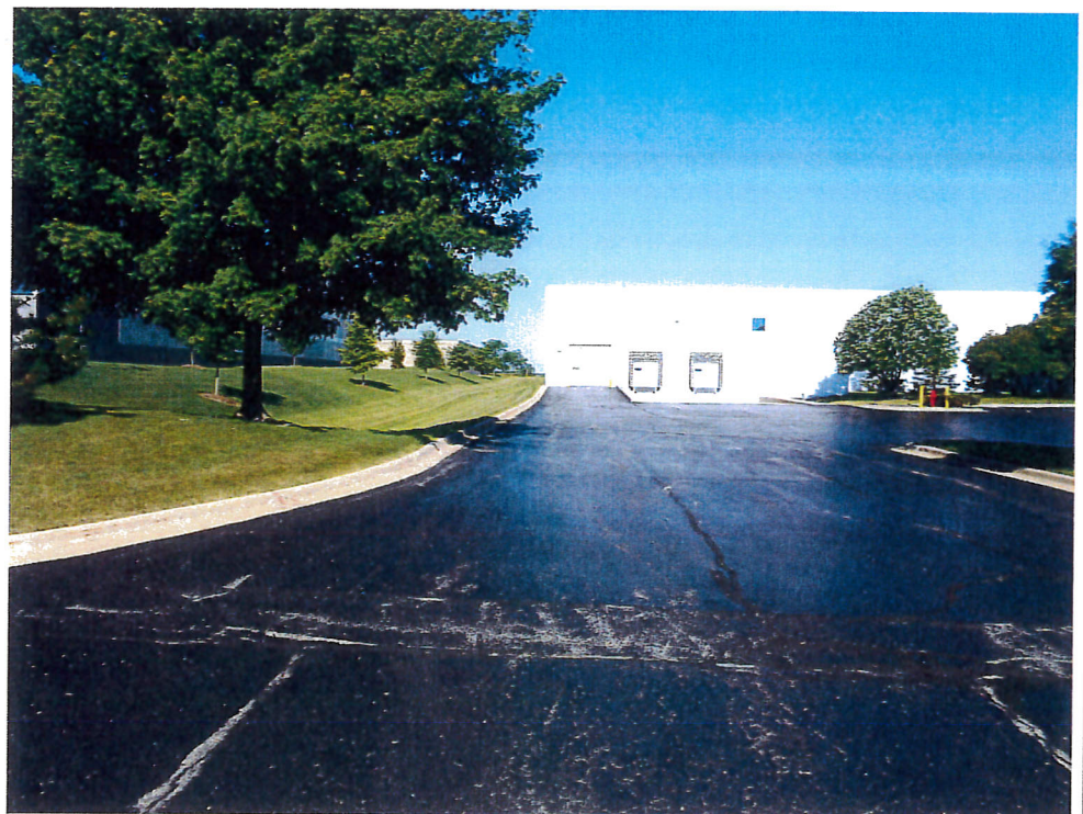
14) View looking west at the south entry drive off of 82nd Avenue. Note the truck docks and the drive-in door at the south end of the warehouse portion of the building.
