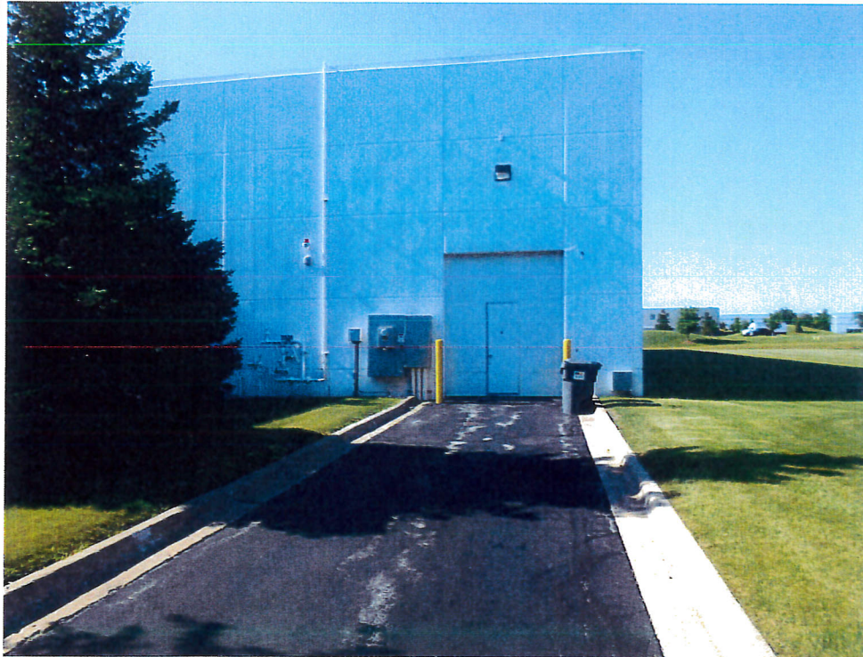
15) View of the second drive-in-door at the west end of the north side of the warehouse portion of the building. The office area is to the left of the photo.
