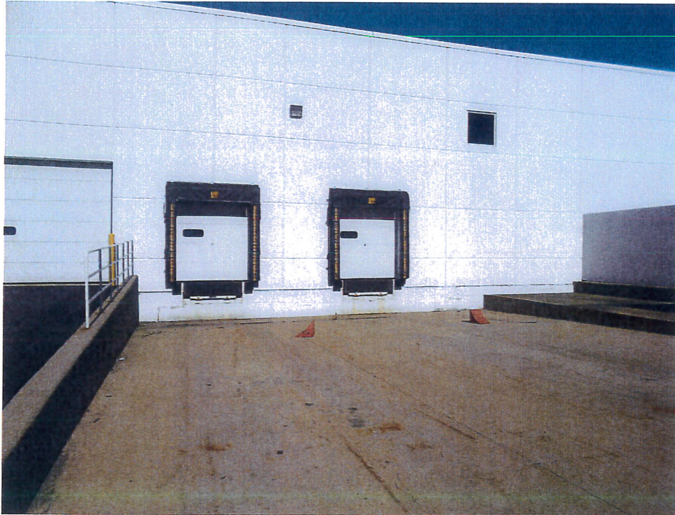
17) View of the depressed truck dock doors and ramp looking west.
